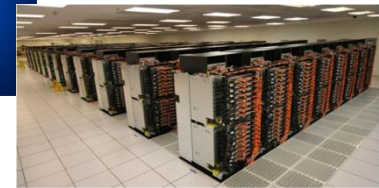
Data centers : AOC
